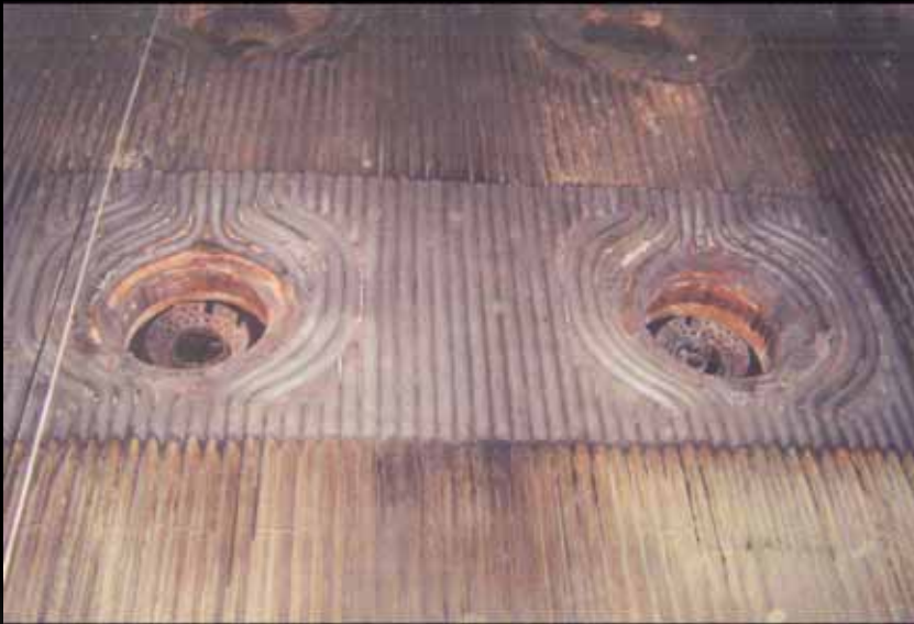
Trial burner grit blast surface preparation
