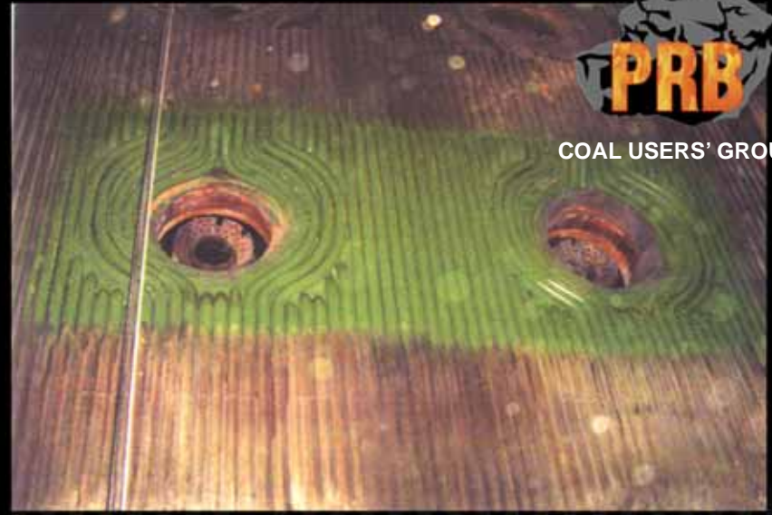
Trial burners with Oxistop MC-19-GR ceramic coating applied
