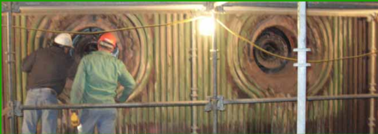
Trial areas (burners) – one year of service slag free
