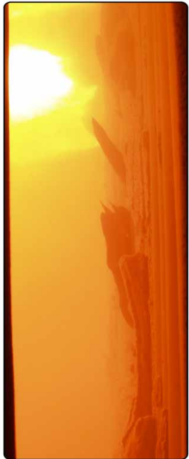
Figure 5 Slag shedding off burner wall coated with Oxistop MC-19-GR on a 192 MW boiler burning 100% PRB coal.
